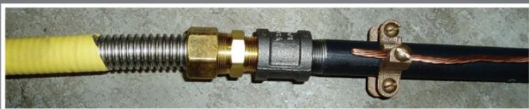
**Check your home for corrugated stainless steel tubing!** Corrugated stainless steel tubing (CSST) is a thin-walled metallic gas piping product that can be used as an alternative to conventional gas piping material or steel pipe. If your home uses corrugated stainless steel tubing, we recommend regular inspections for your safety and to prevent potential dangers and code violations.
